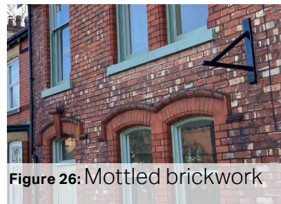
Figure 25: Brick and stone archway above door
