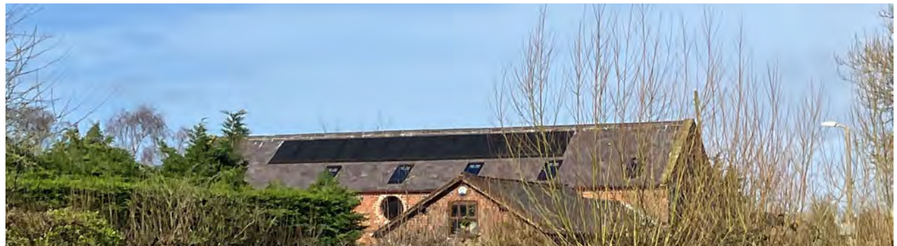
Figure 54: Solar panels on a converted farm building along South Road
