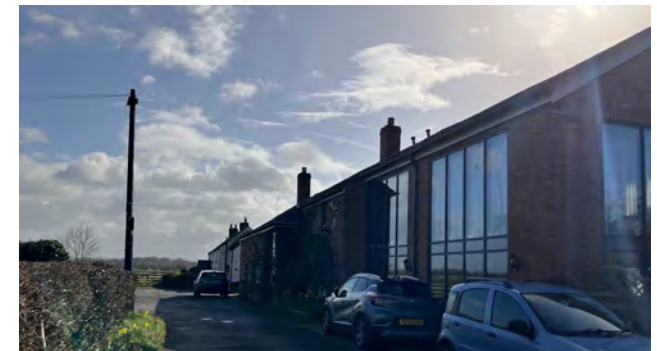
Figure 16: Converted and extended agricultural buildings
